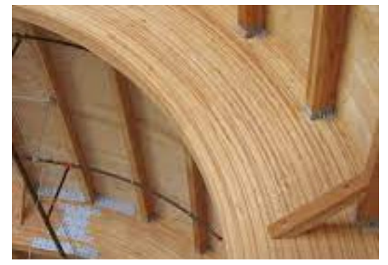
Custom Curved Glulam Columns
